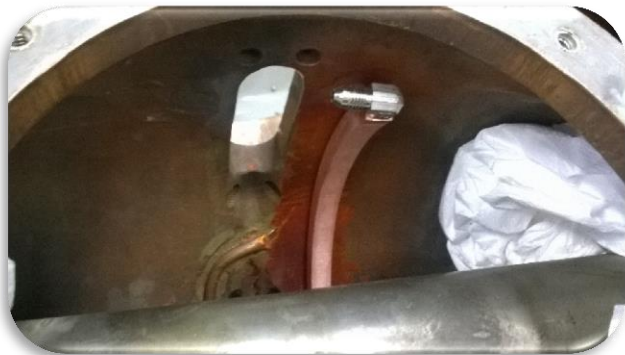
Water cooling repair/upgrade
